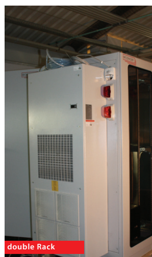
IT security cabinet / 19" gas extinguishing system
